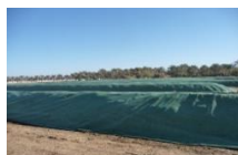
composting facility Royal Court Oman
