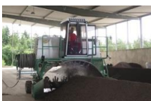
indoor composting facility Germany
