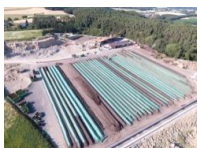
composting facility Austria
